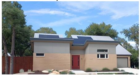
**The 1025 Lane Street residence** is a high performance zero energy building combining solar energy, ground source heat pump HVAC, an envelope with a ventilated metal roofing system, a ventilated wall system, a motorized insulated interior shading system, appoint controlled LED smart lighting, rainwater collection, and xeriscaping. This building generates 750 kWh more energy than it consumes from the grid every month, allowing the owner to sell power back to the grid.
